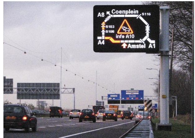
Information board displaying the location of congested traffic in red on the ringroad of Amsterdam (Source: Trinité).
