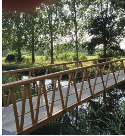
This footbridge (Nederwetten, The Netherlands) is made of more steel than strictly necessary to assure its quality. Software engineers must also consciously employ redundancy to ensure quality.
